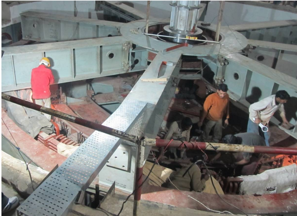
Figure 67: Hydrogenerator under construction
