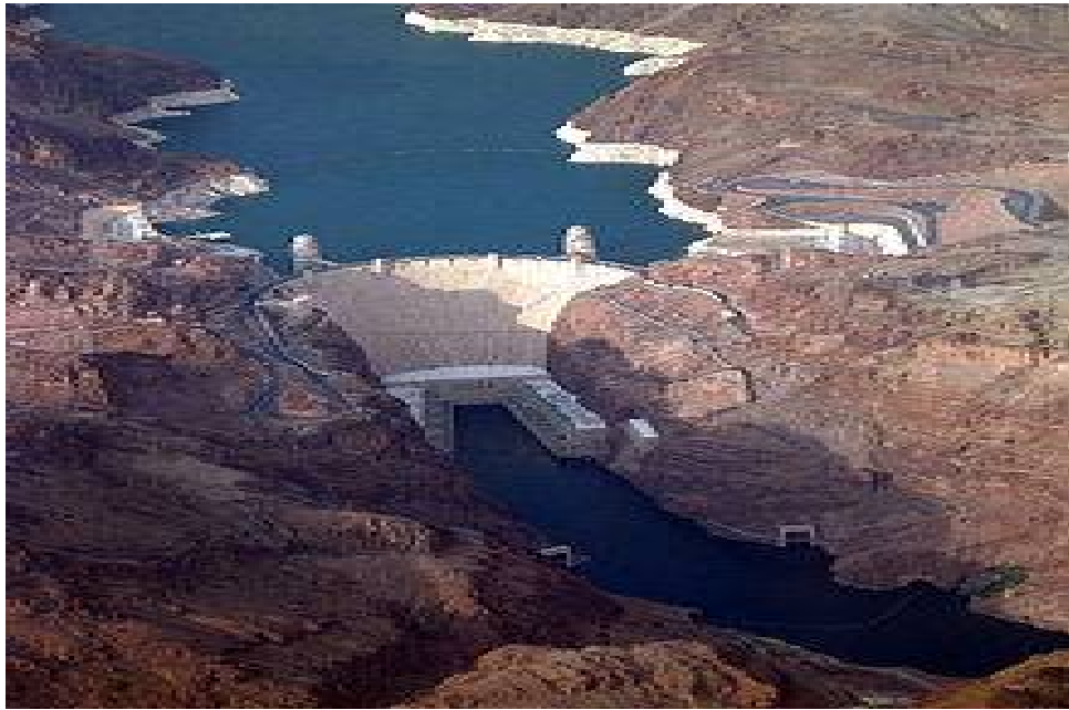
Figure 8: Arc Gravity Dam
