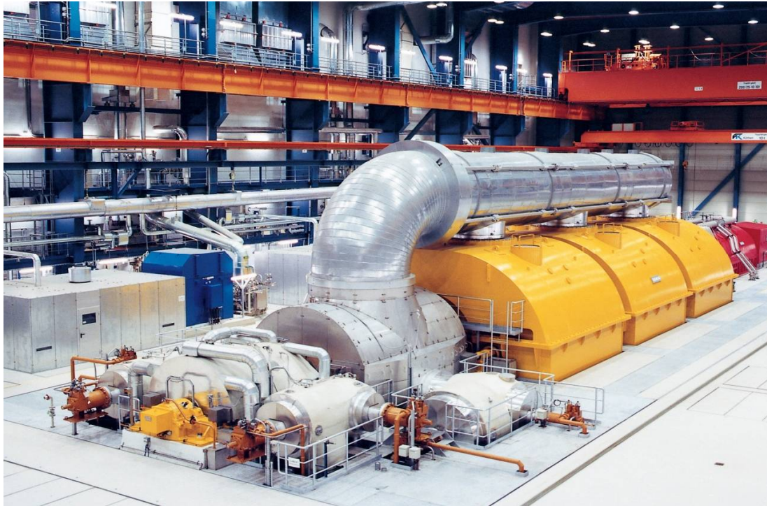
Figure 69: Turbogenerator
