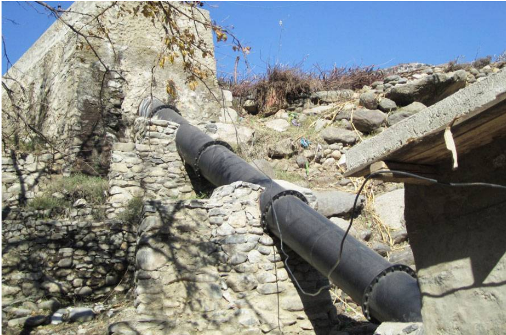
Figure 11: Forebay with Penstock
