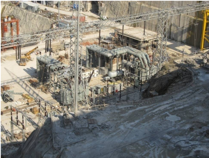
Figure 18: A switchyard under construction
